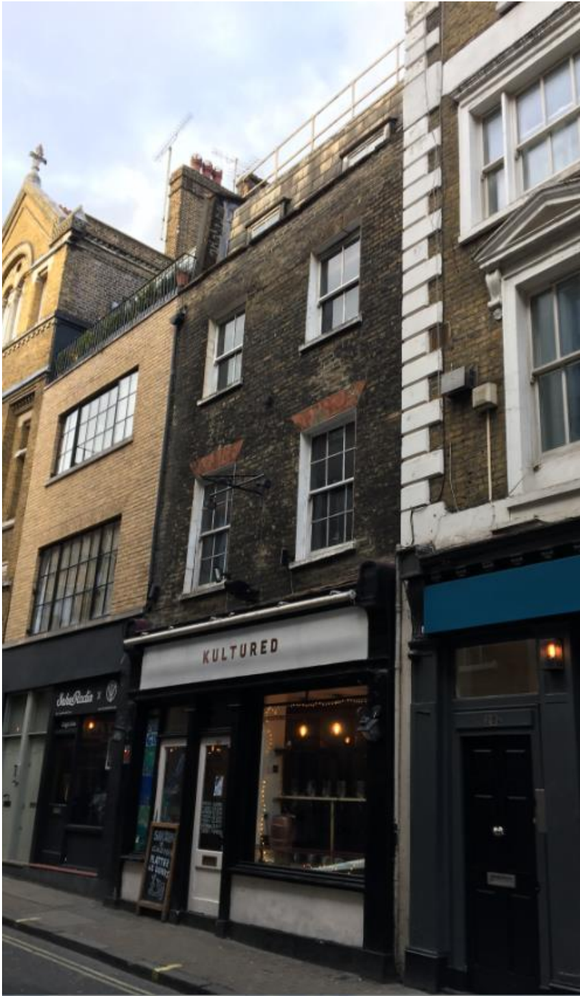
Front elevation of building:
